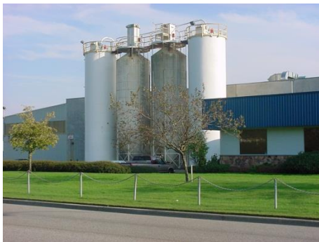
Ipex Plant on Duncan Way
